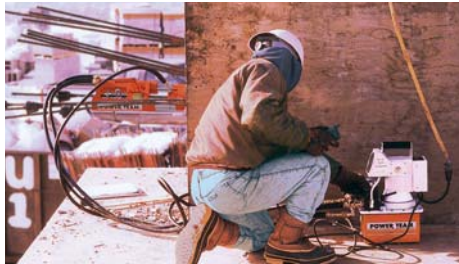
The PE60 used for pre-stressing.
